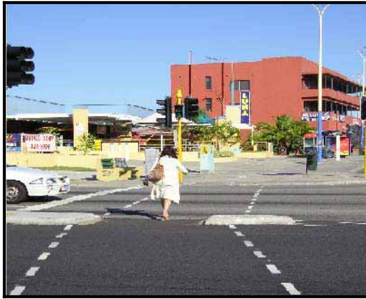
Photograph 15: Marked foot crossing
